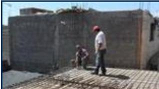
Past. Marcos & Bro Nelson placing rebar, part of the 2<sup>nd</sup> floor support.
